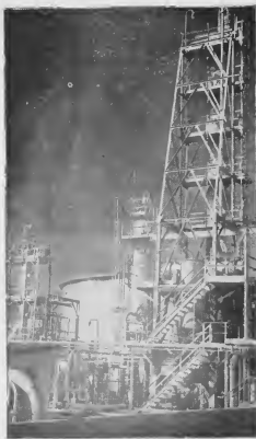
Propane is extracted from refinery gases in the tall towers at right. The smaller unit at left takes moisture from the product before it is stored.
